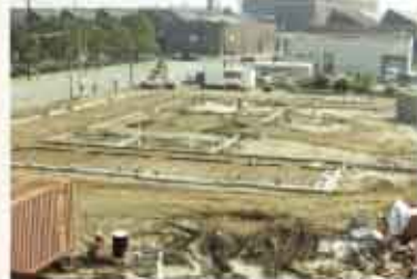
Construction of Pathways
